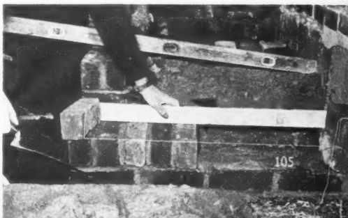
Above: Making an outside wall for steps. Bricks should be wet for best results. Below: Aligning the first step. A level, straight edge and string—plus a bit of patience—will produce a good looking and lasting job.
